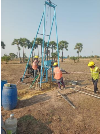
fig-8 Retrieval of samples
