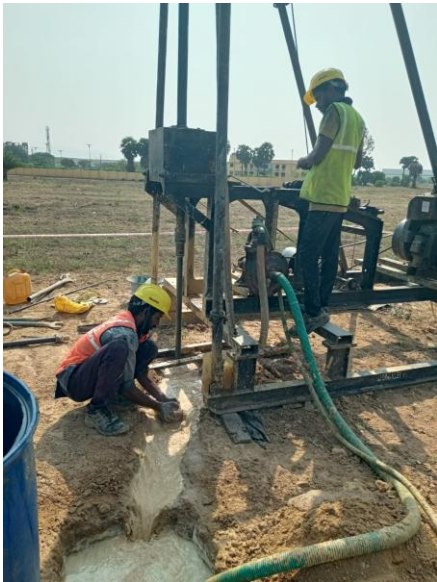
fig-2 Borehole drilling
