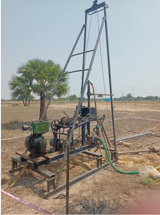
fig-4 Drilling Rig
